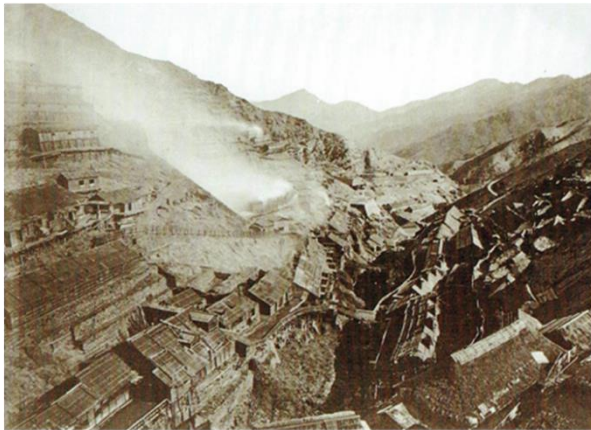
Photo 5 Besshi Copper Mine before foresting (1881)
